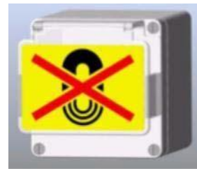
Scan room quench button located behind door
